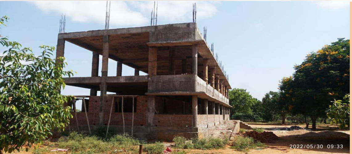
Construction of New Classrooms Block
